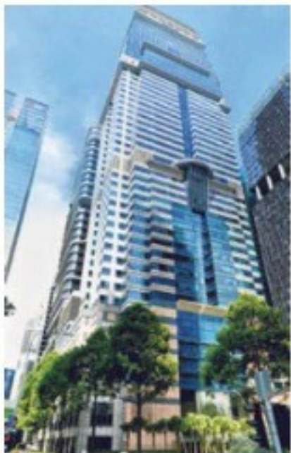
operational at Asia Square Tower 2 ght: ByteDance is in talks to lease gan at Capital Tower in
